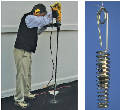
The membrane is protected from coming in contact with the soil by a wire hanger.
